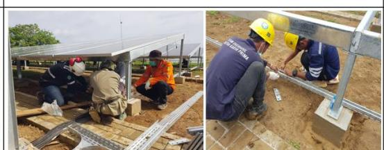
Wiring Cable DC PV Panel to Inverter
