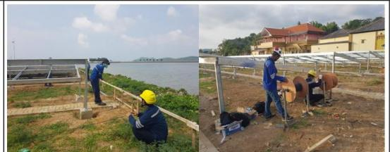
Wiring Cable DC PV Panel to Inverter
